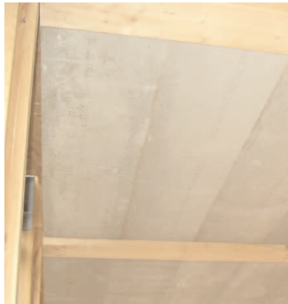
Cetris board ceiling, Upton, Northampton
