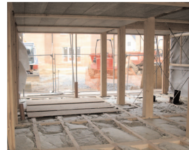
Insulation in ground floor at Upton, Northampton
