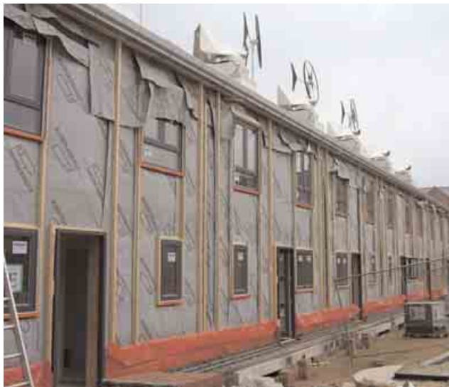
The 'air tight box' at Upton, Northampton
