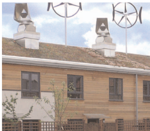
Timber cladding at Upton, Northampton
