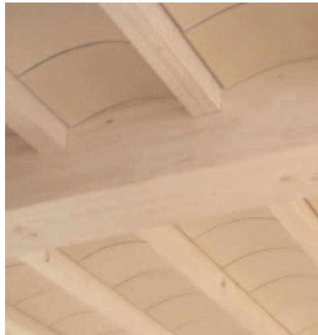
Ibstock floor bricks at Eco Build Show House
